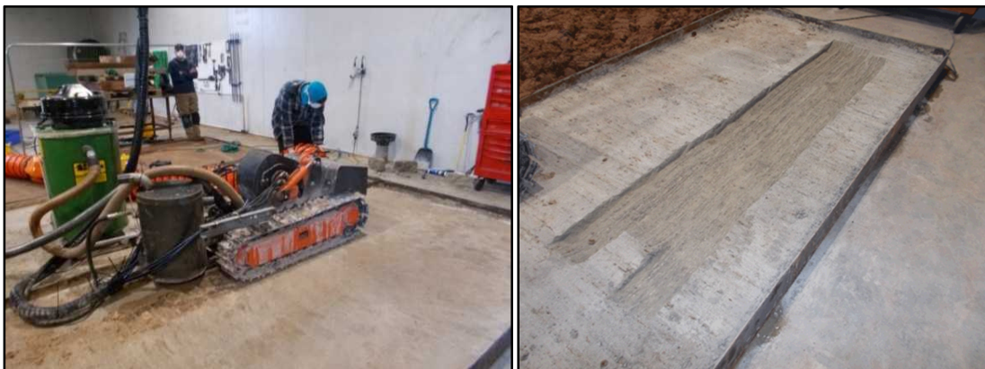
Figure 9. Robotic Crawler with Rotocutter and Retrieved Simulant.
