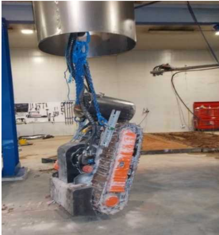
Figure 10. MWGS Deployed through a 42-in. Opening.
